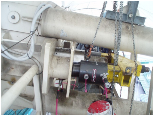
Figure 2: Jacking equipment
