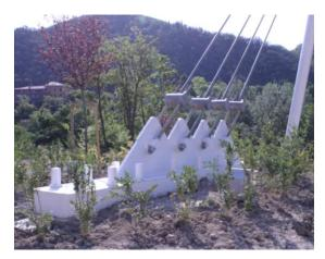
Fig.5 View of the suspended footbridge over the river Reno (left) and the anchoring support (right)
