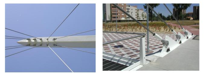
Fig.8 Upper anchoring of front cables (left) and lower anchoring of back cables (right) of the stayed bridge over the river Reno
