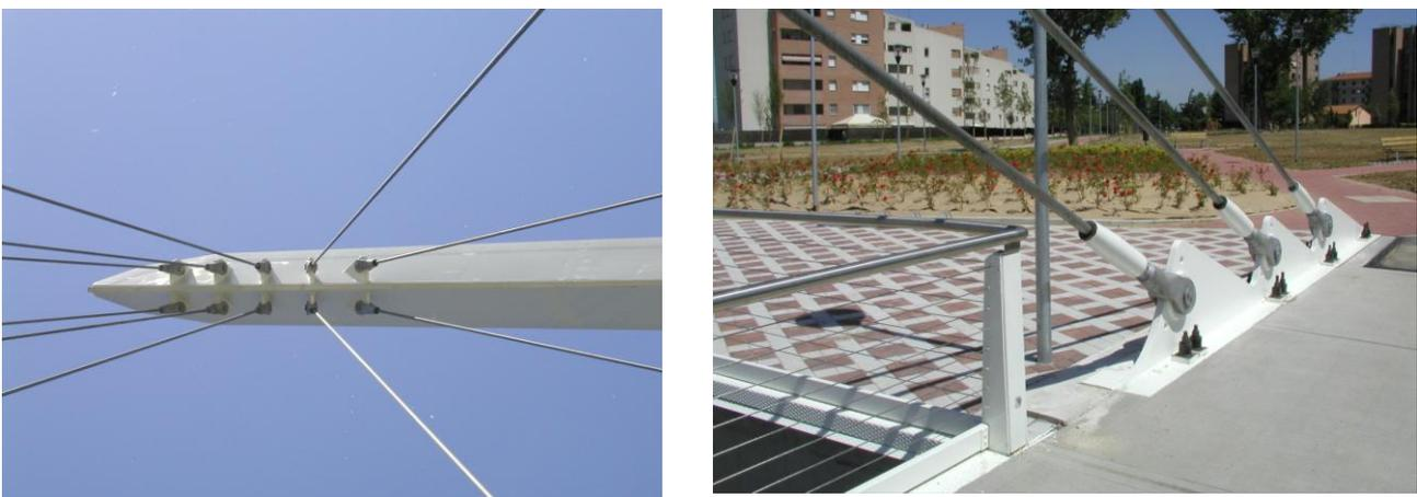
Fig.8 Upper anchoring of front cables (left) and lower anchoring of back cables (right) of the stayed bridge over the river Reno
